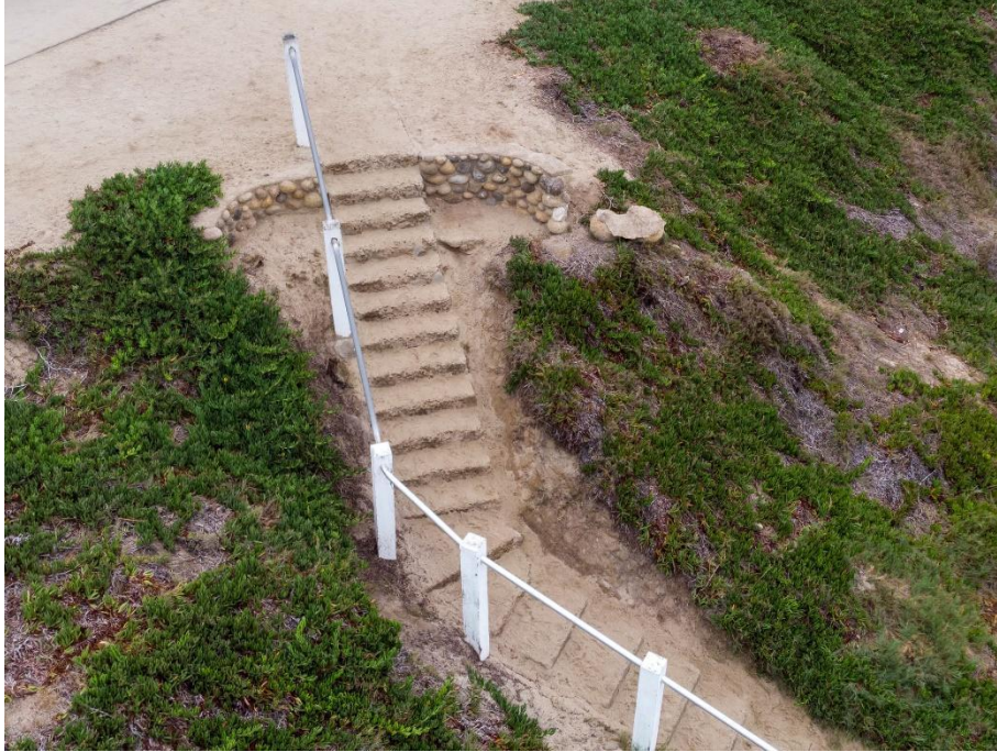
Photo 33 Whale View Point Stairs, camera facing south
