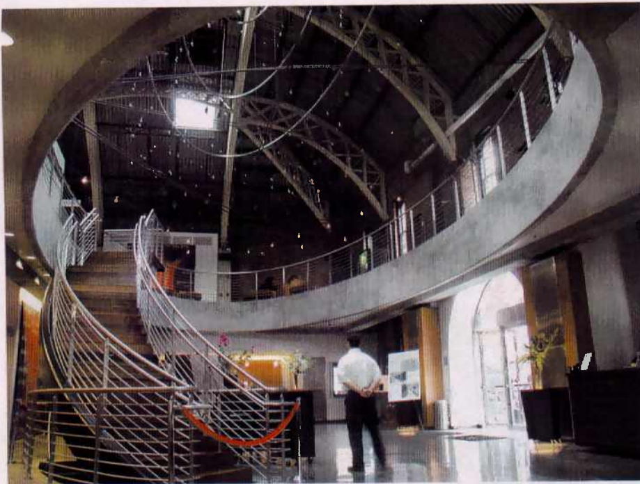
In one of the boldest moves in the interior, the armory renovation team designed a large oculus in the second floor that preserves views from the first floor to the building's historic wood roof trusses. Other sustainable elements included new skylights for natural daylighting, which were actually part of the building's original design. Photo: courtesy of Green Building Services
