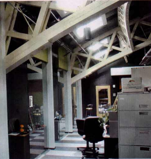
Above: Massive trusses hewn from old-growth wood are among the most character-defining elements of the historic 1891 building and were carefully preserved even in the tricky modern office spaces. Photo: courtesy of Green Building Services
