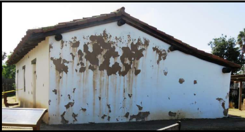
Figure 8: An Illustration of How Quickly Adobe Buildings Can Obtain an Unkempt Appearance. The peeling plaster on the Machado-Stewart House (left) and the Rodriguez Adobe (right) in Old Town San Diego State Historic Park are the results of heavy winter and spring rains in 2023. These buildings are constantly maintained by California State Parks (Photograph by Stephen R. Van Wormer).
