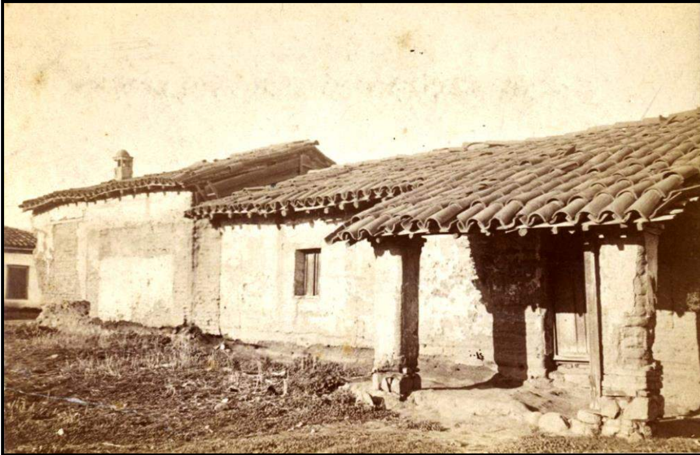
Figure 9: 1884 Photograph of the Teodoro Arrellanes Adobe in Santa Barbara. This image illustrates what can happen if constantly peeling plaster, as illustrated in the previous figure, along with erosional deterioration at the base of the walls caused by water seeping up through the blocks from the ground, is not repaired. The result is the perceived unkempt appearance of adobe buildings to observers not accustomed to the characteristics of adobe architecture (California State Library; https://delivery.library.ca.gov:8443/delivery/DeliveryManagerServlet?dps_pid=IE210737 ).
