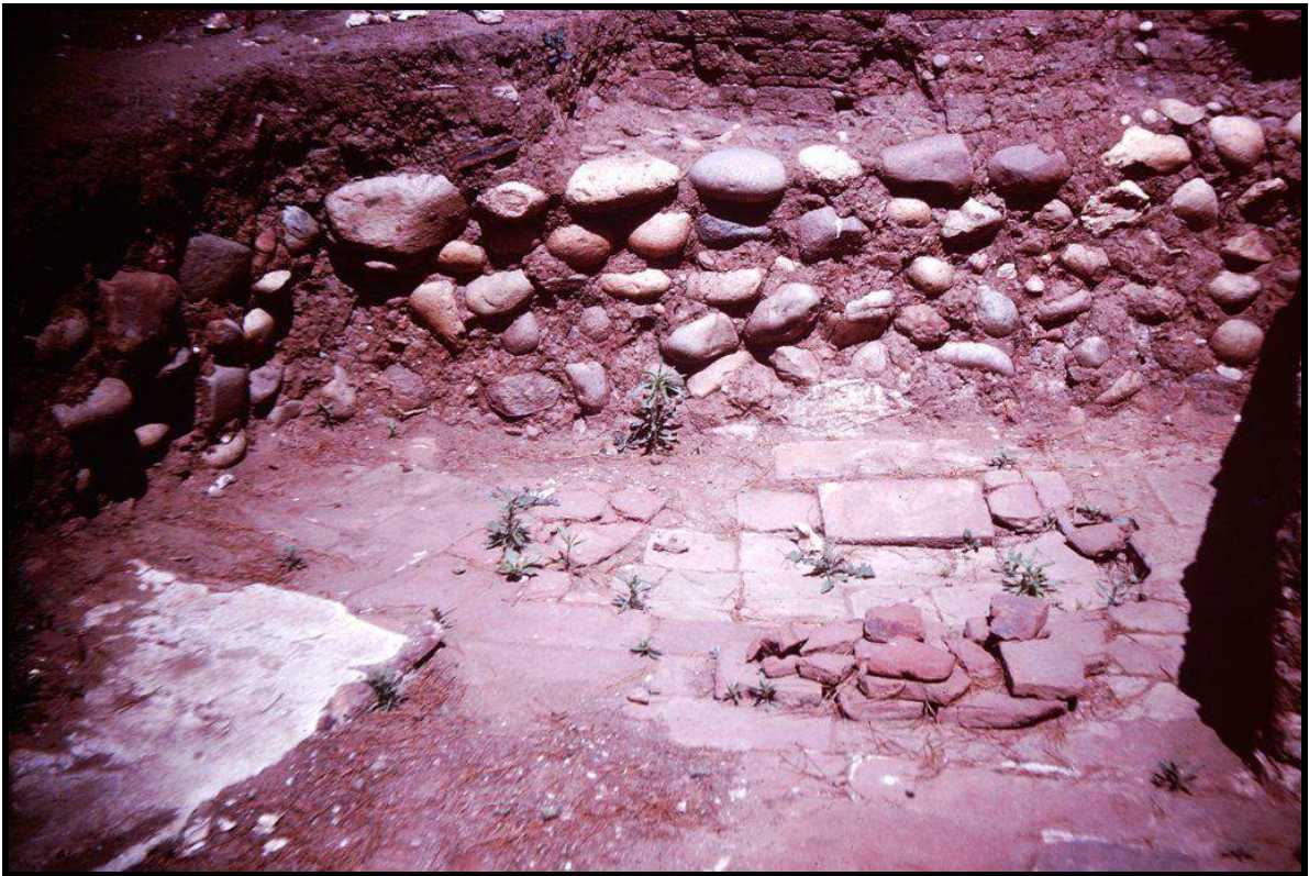
Figure 7: Typical Chapel Construction Detail. Cobblestone foundations support the remains of adobe block walls, which can be identified in the photograph by the horizontal mortar joints between the blocks. Ladrillo tiles cover the floor. The photograph was taken in the side chapel looking toward the northeast (Courtesy Stan Berryman).
