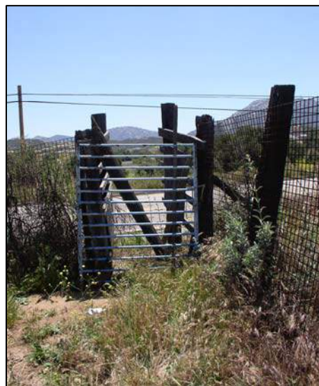
Blocking gate to restrict cattle access.
