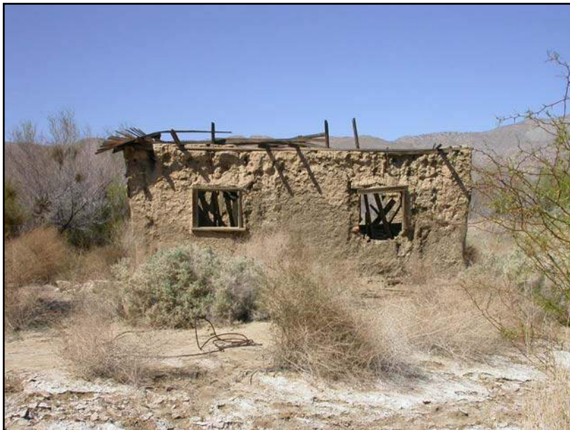
Bailey earthen structure - 2003
