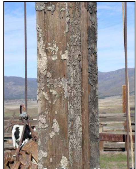
Tar covered upright made from bridge salvage material.
