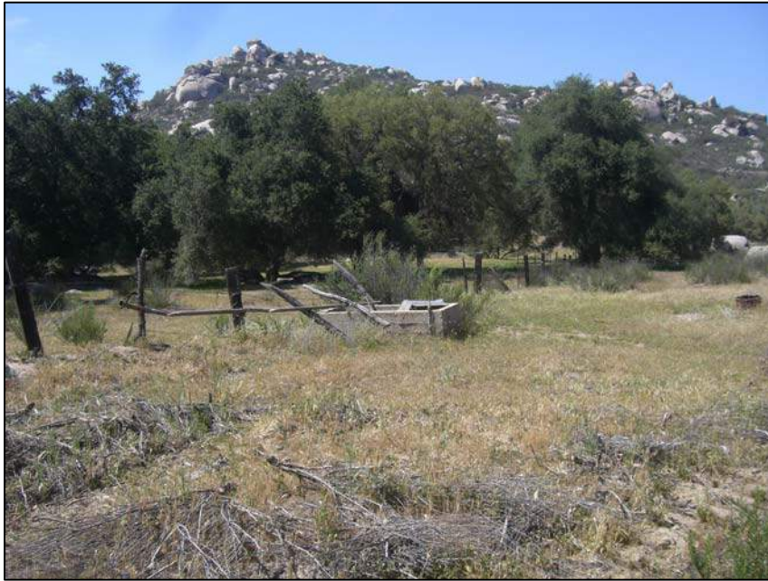
Concrete trough at Round Potrero.
