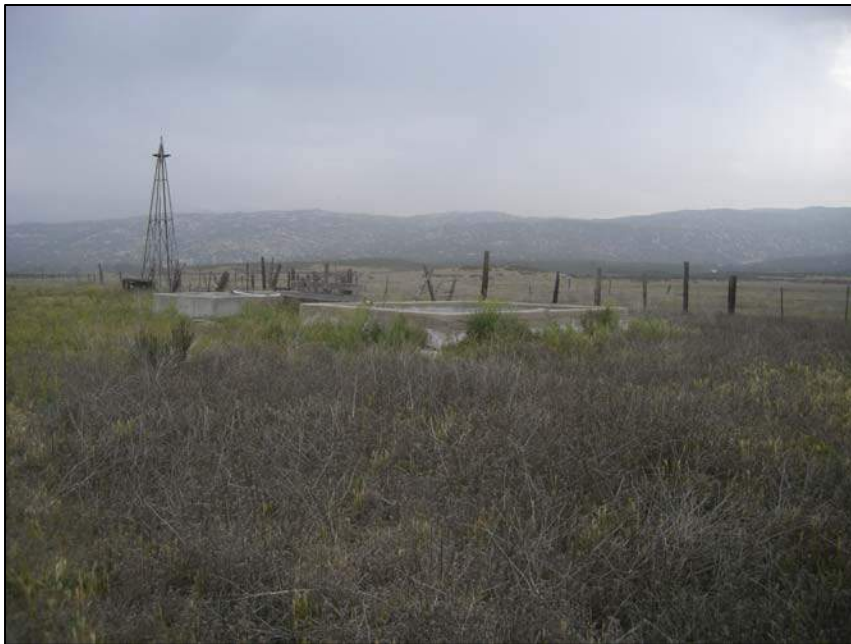
Windmill and concrete reservoirs in Long Potrero.
