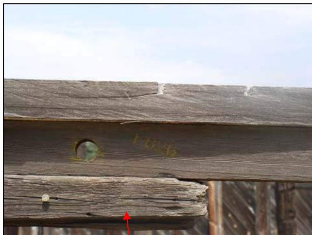
Power pole used as horizontal beam.
