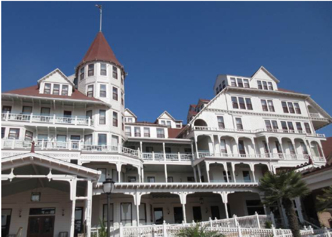
Figure 82: After - Same view after restoration, 9-13-21.
