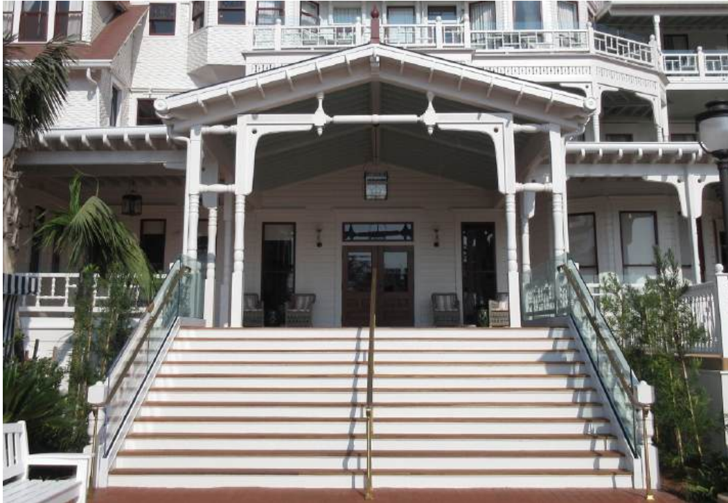
Figure 48: The main entry stairs include replicated 1888 wood spindle handrails and newel posts, all custom made from mahogany. Frameless glass guardrails and a center bronze handrail were incorporated to comply with code requirements.
