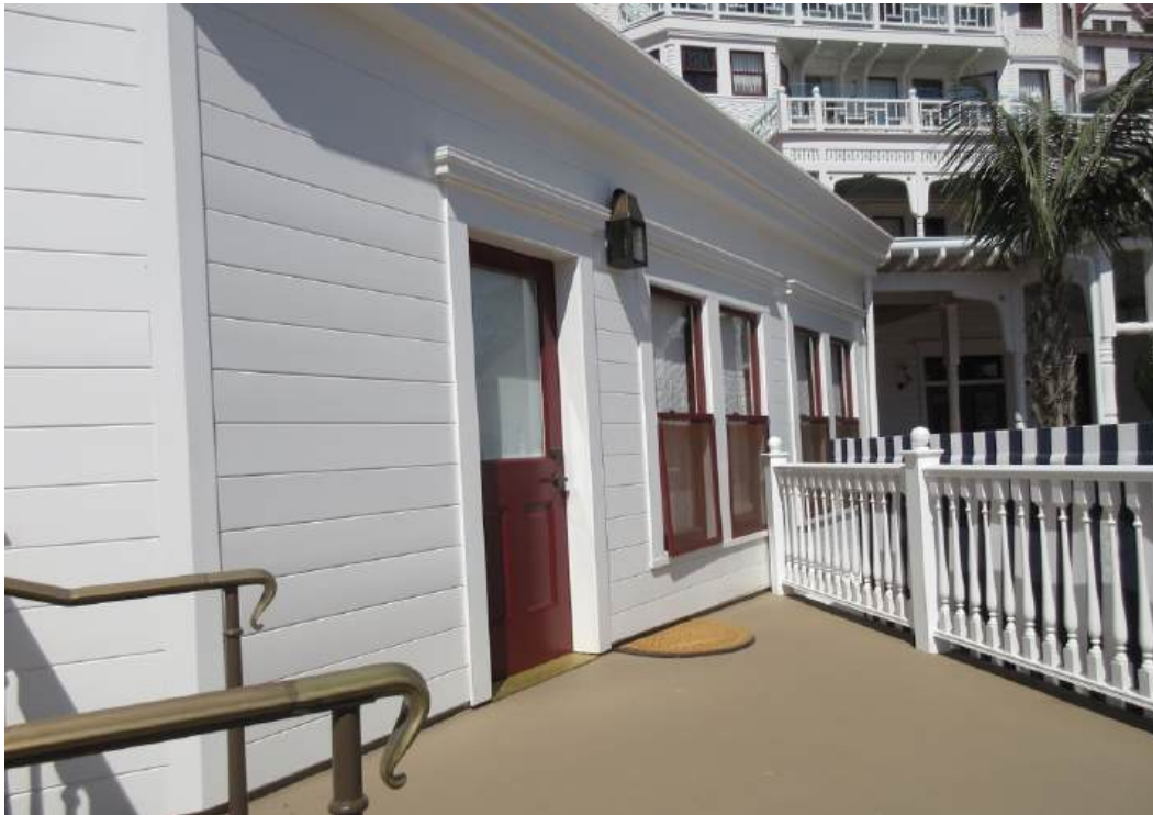
Figure 55: The exterior wall of the General Manager's Office is part of a ca.1930s addition to the Ballroom. This façade was remodeled to better coordinate with the restored Veranda. Faux columns were removed and four new windows and a door were added. The horizontal V-groove siding, cornice, door and picket railing differentiate this façade from the historic facades.
