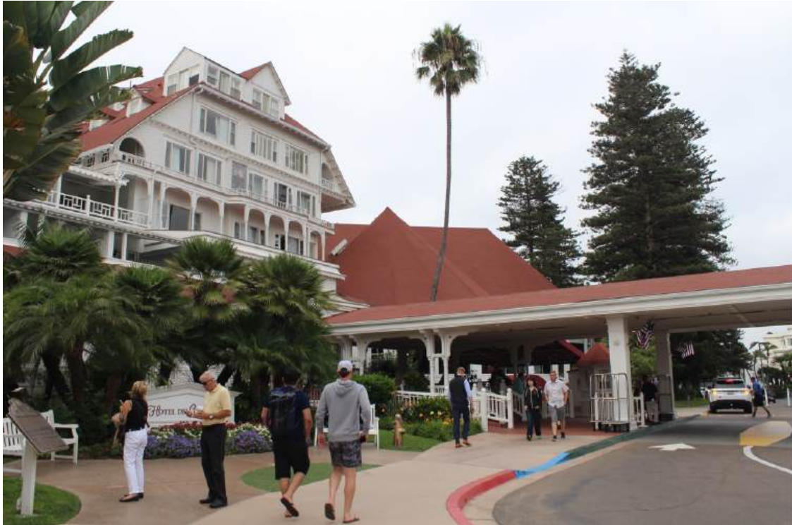
Figure 79: Before - View of the south façade and Porte Cochere looking northeast, 9-24-18.
