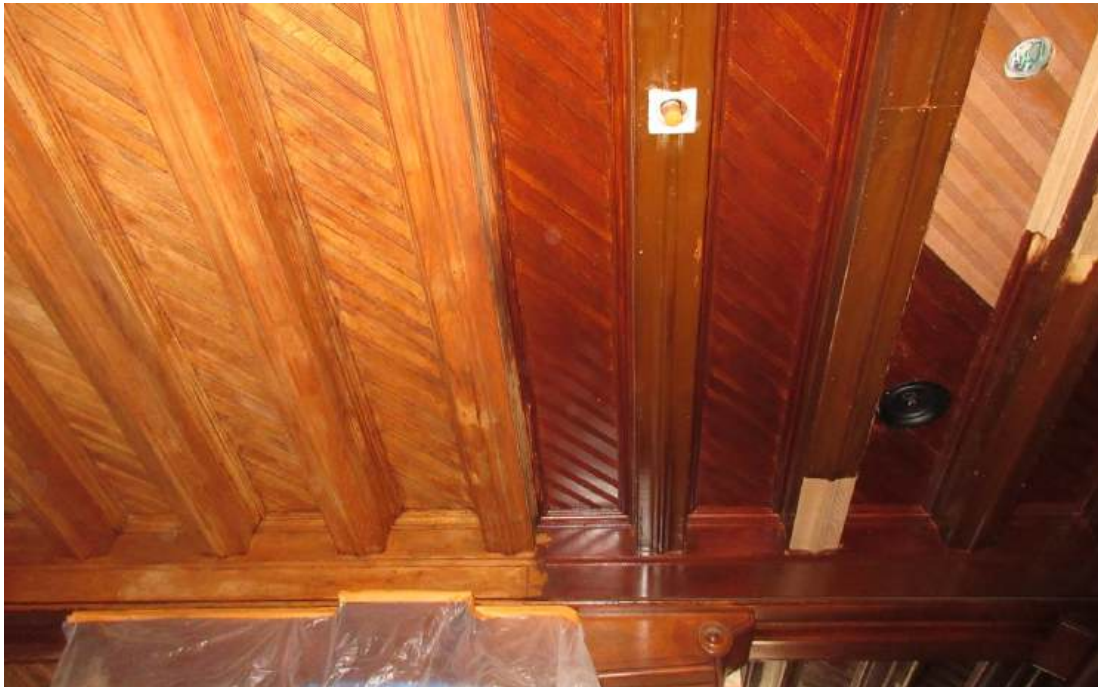
Figure 27: Much of the Lobby woodwork had been painted and/or re-stained (right). The ceiling on the left shows the white oak after being stripped, prior to the application of new stain and shellac. The lightest areas show where new oak was used to patch missing or damaged pieces.
