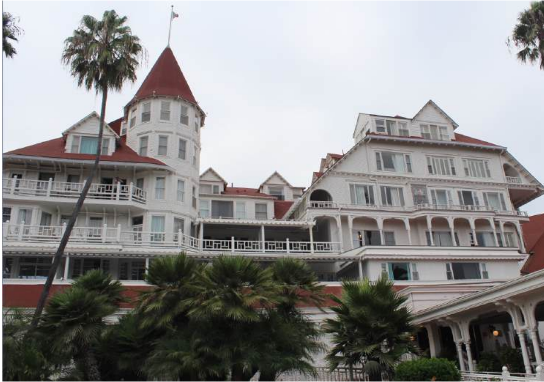
Figure 81: Before - View of the upper south façade, 9-24-18.
