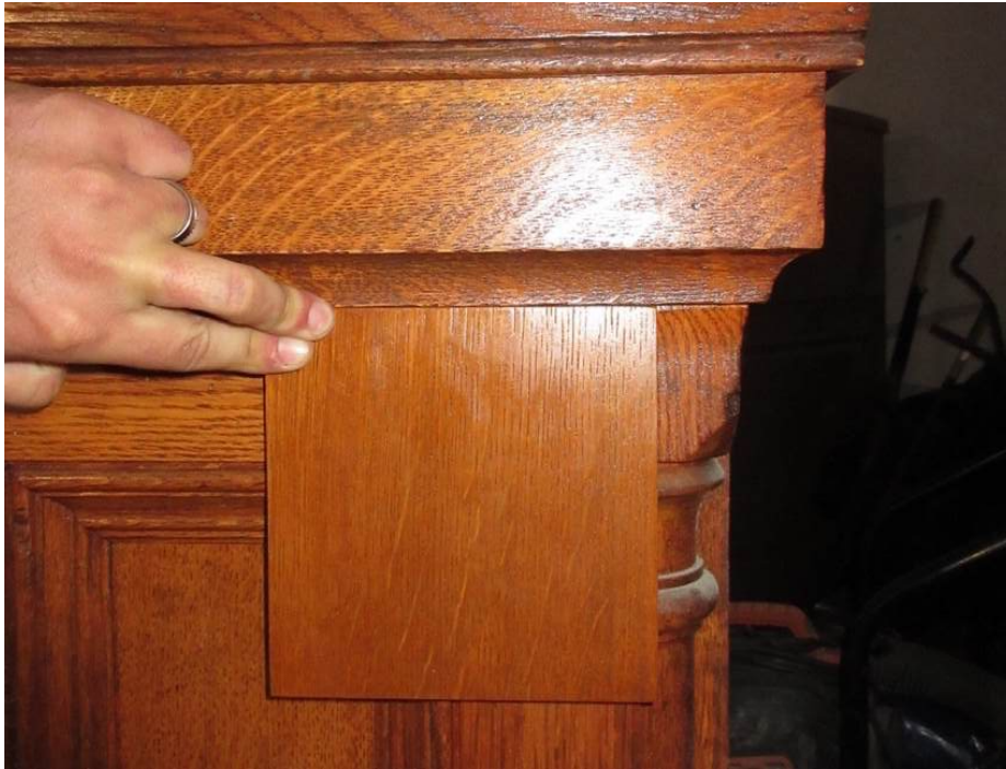
Figure 28: Matching the historic “golden oak” wood finish at an original Lobby column.
