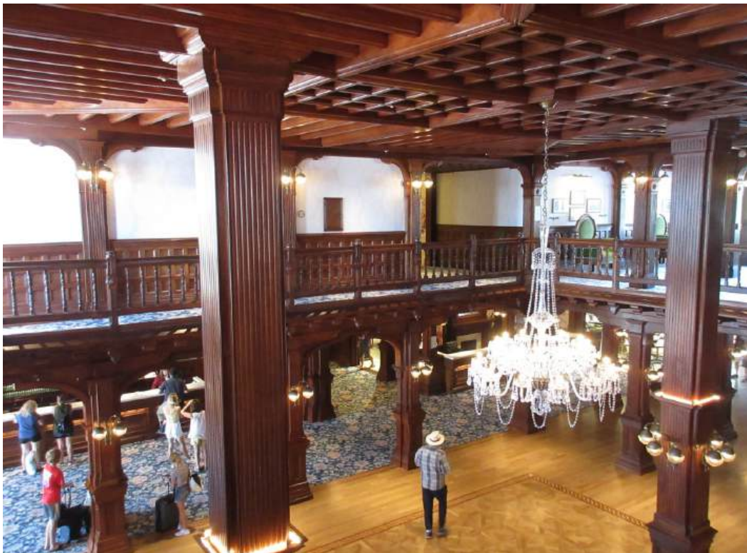
Figure 96: After - Same view after restoration, 9-23-21.
