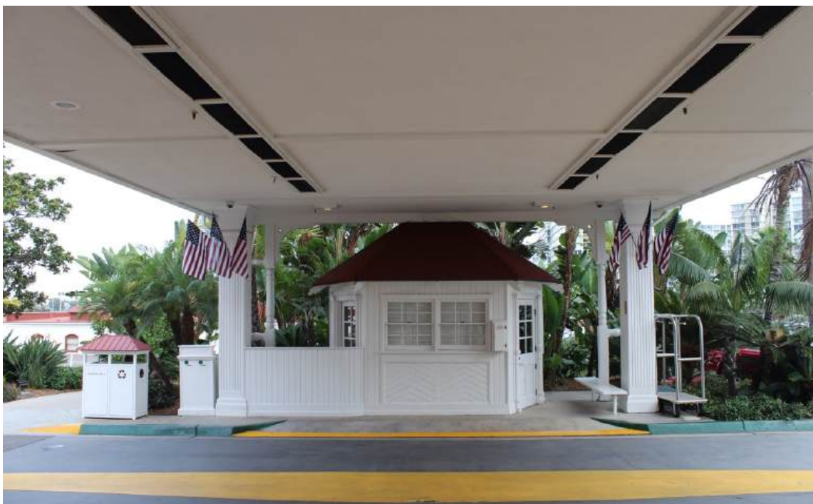
Figure 10: View of the 1979 Porte Cochere with flat stucco ceiling and oversized square posts. The VIP Check-In is the free-standing pavilion.
