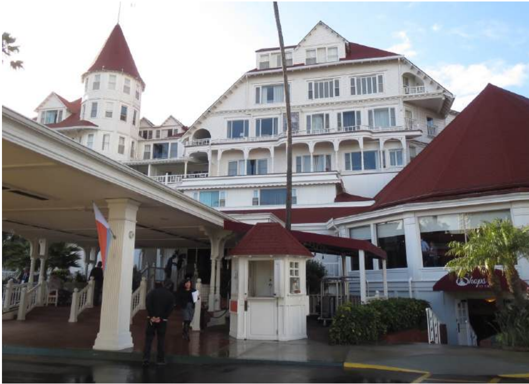
Figure 83: Before - View of the east end of the south façade, 2-27-18.
