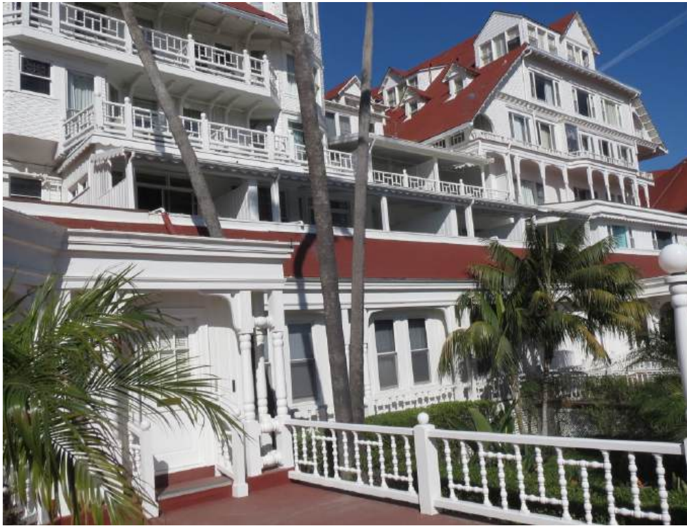
Figure 85: Before - The west end of the south façade from the General Manager's deck, 1-25-18.
