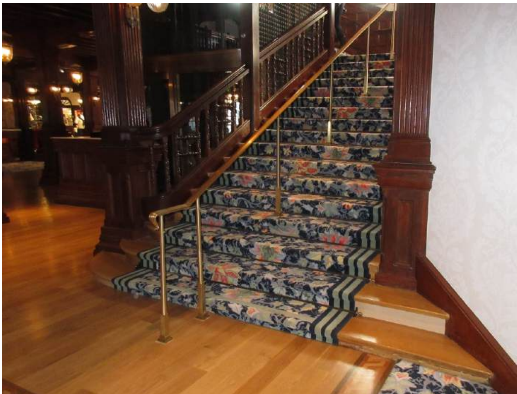
Figure 37: The main stairs in the Lobby after repair of the damaged treads. A new carpet runner and center bronze rail were installed.
