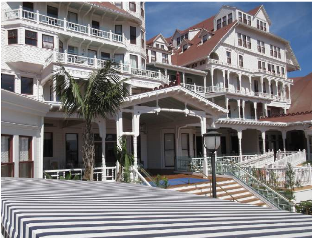
Figure 86: After - Same view after restoration, 9-23-21. The luggage cart canopy is in the foreground.
