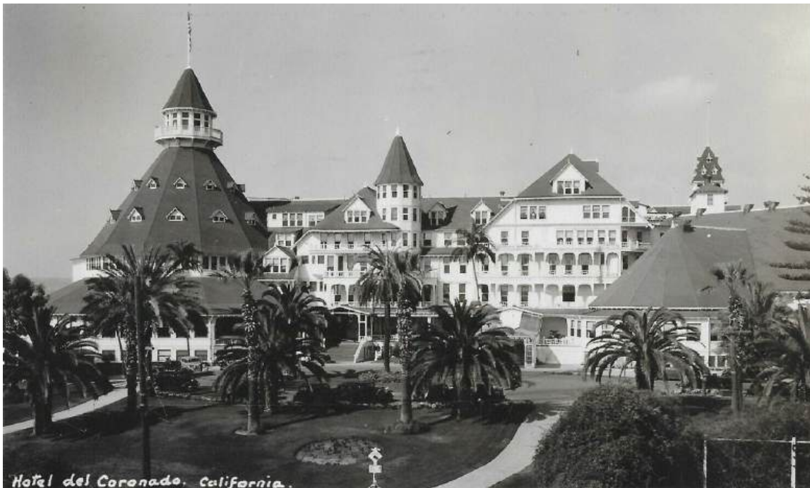
Figure 4: Historic postcard of the south façade, ca.1935. Note the missing grand chimney and added upper floor windows. Image credit: David Marshall Collection.
