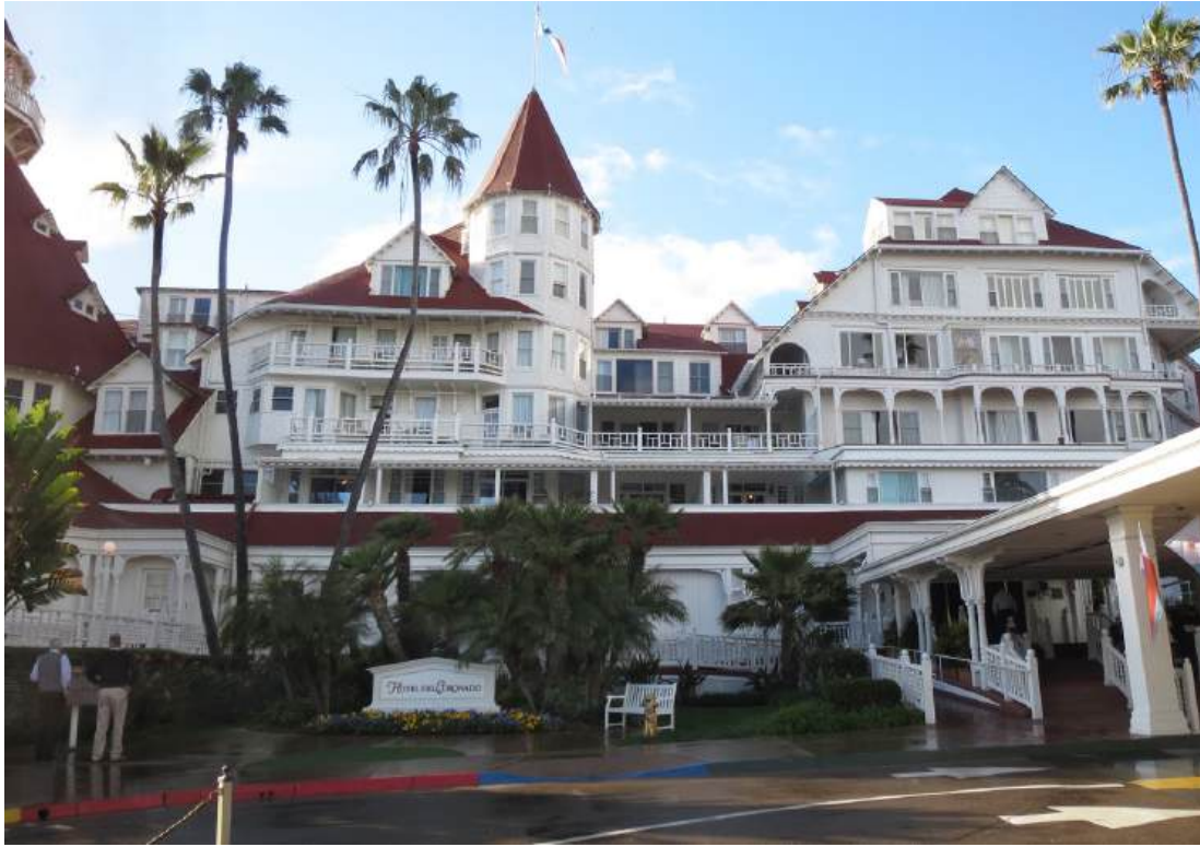
Figure 77: Before - View of the south façade, 2-28-18.
