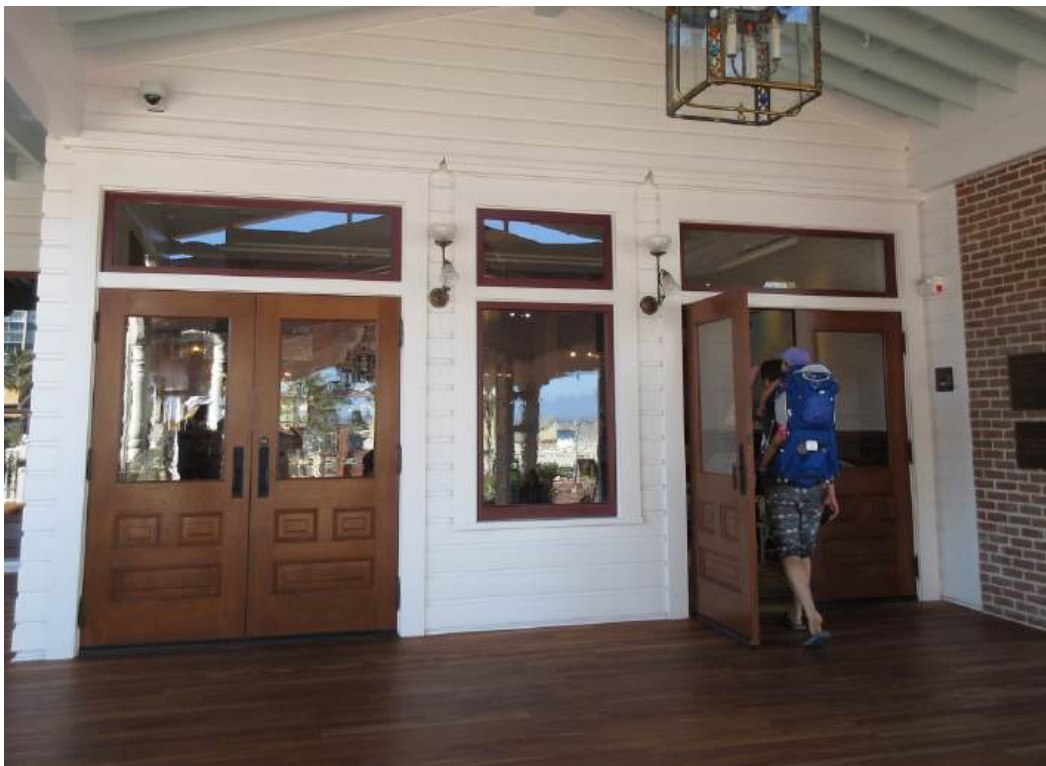
Figure 90: After - Same view after restoration with two historic door pairs recreated, 9-19-21. The three stained-glass transoms still need to be installed.
