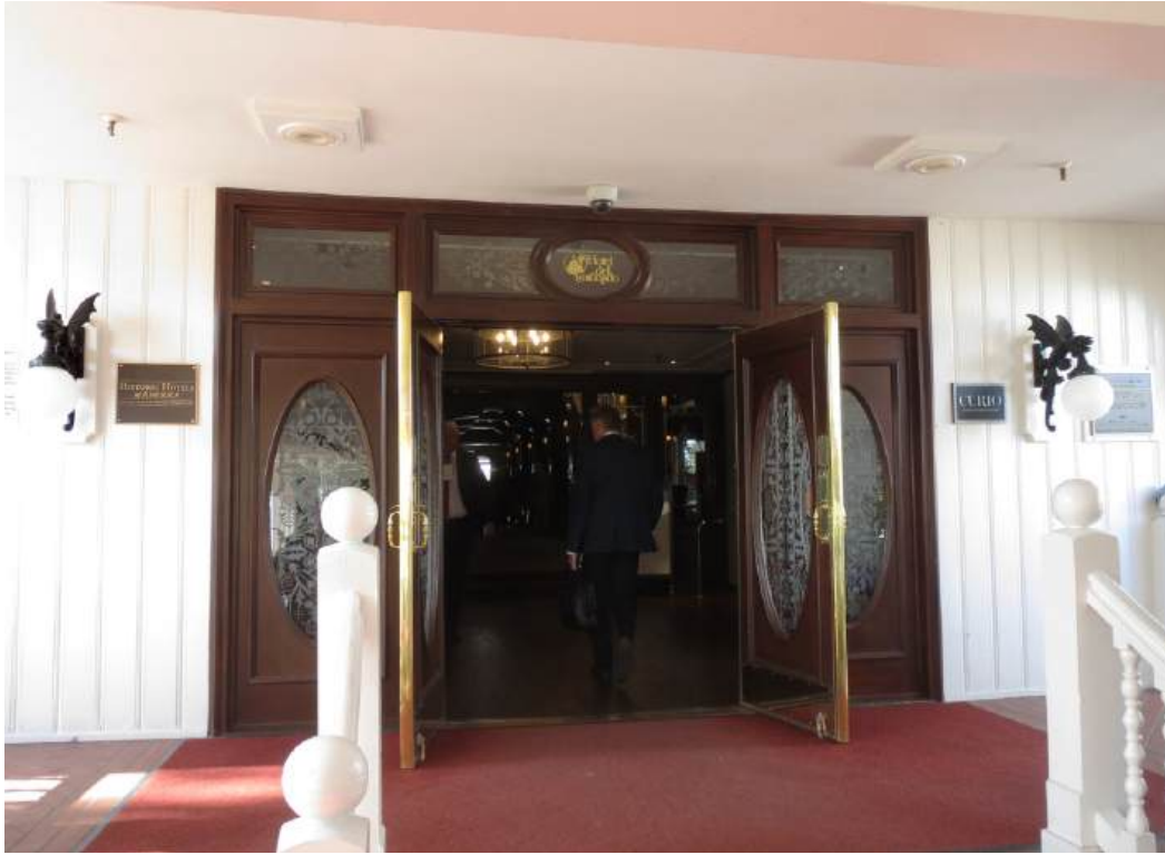
Figure 89: Before – The non-historic ca.1980s entry doors and gargoyle sconces, 2-27-18.
