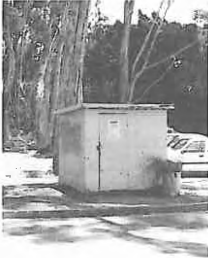
An existing grounds maintenance shed.
