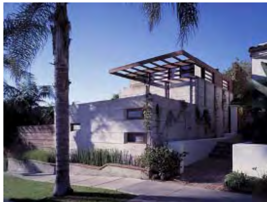
Rudolph Schindler's Pueblo Ribera Court, 1923. Schindler's slipform concrete construction technique resulted in the visible horizontal lines in the wall plane. Courtesy www.mosslerdoe.com .
