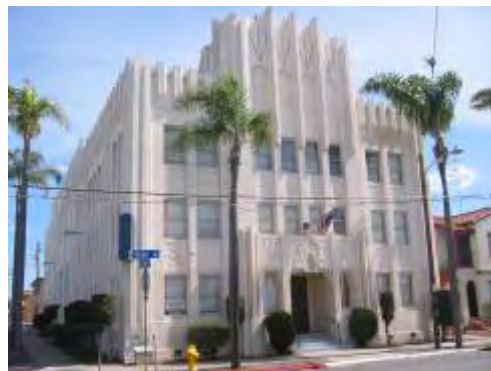
The Masonic building in North Park demonstrates an Art Deco style symmetrical façade, as well as vertical massing and fluting, and zigzag details.
