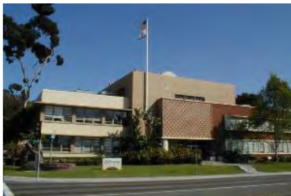
Caltrans building in Old Town, designed by CJ Paderewski in 1953. Note the horizontal bands of windows accented by a plaster surround.
