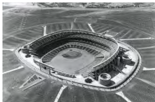
Construction and completion of the San Diego Stadium by Frank L. Hope & Associates. Courtesy of the San Diego Historical Society.
