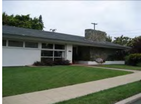
A Custom Ranch home in Mission Hills. Note the horizontal roofline with deep overhangs and linear arrangement of windows. This house also features a prominent stone chimney and a generous front yard, both typical features of Ranch style homes.
