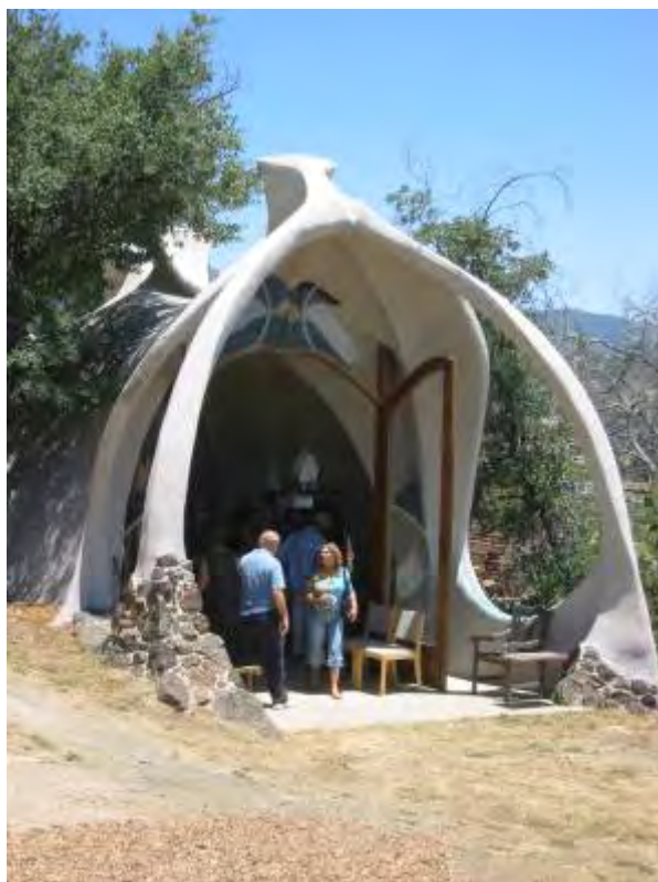
The Hubbell compound in Santa Ysabel by James Hubbell work on this site has been ongoing since 1958. The compound includes several structure holding the Hubbell’s home, studios, and galleries. This photo shows the studio.
