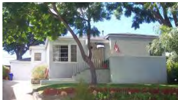
This Minimal Traditional residence located in Rolando features a combination of stucco and wood siding exterior finish materials, Moderne inspired corner windows and a detached rear garage.
