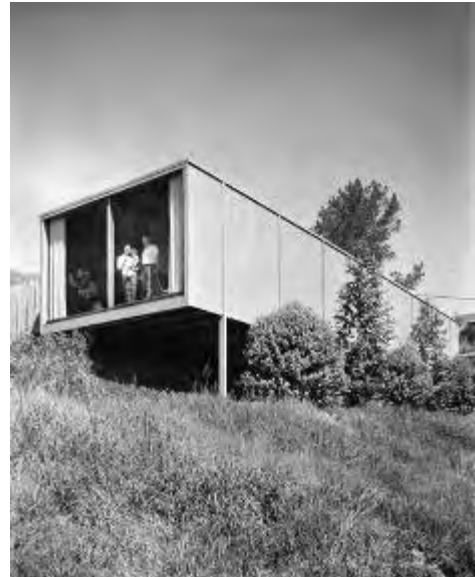
The Boxcar House in Mission Hills, designed by Homer Delawie in 1958. The 16-foot wide home was built on a steep narrow lot. The lack of roof overhangs (a typical Delawie detail) accentuates the boxy form. Courtesy of Douglas Simmons.
