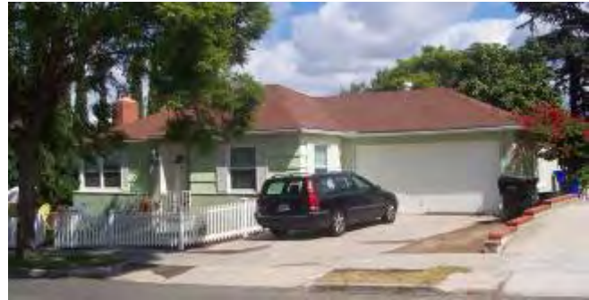
Located in Rolando, this Tract Ranch residence exemplifies mixing of traditional architectural details such as horizontal wood siding, wood shutters and a brick chimney with modern conveniences such as the attached two car garage..
