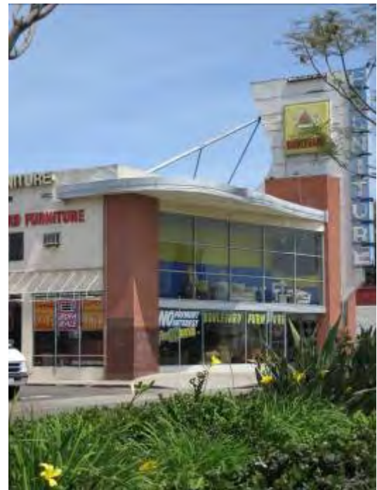
Dennstedt Electro Mart, built ca. 1941 (now a furniture store). The building exhibits aspects of early Modern and Googie architecture. Note the prominent signage, curved roof projection, and large aluminum storefront windows.
