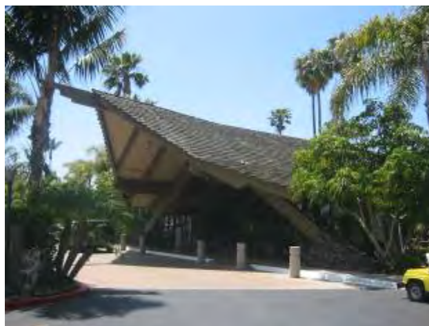
Shelter Island Hotel was designed by Richard Wheeler in 1960. Note the wide cross-gable marking the front entry and the heavy timber construction, which includes a large A-frame roof that continues to the ground. This building also features a tropical landscape and strong horizontal massing. The primary exterior materials include wood and stone.
