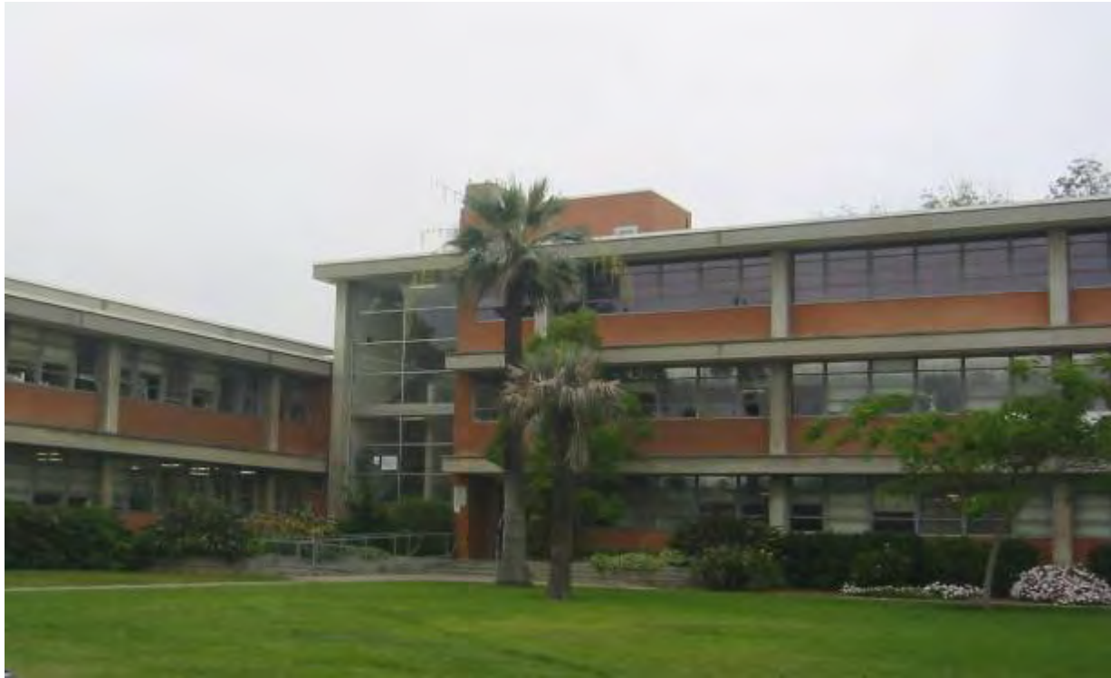
Education Center in University Heights, designed by Clyde Haufbauer in 1953. Note the horizontal bands of steel sash windows, the strong horizontal roof line, and the use of brick between the concrete frame to accentuate the linear structure.
