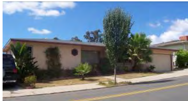
This example of a Tract Ranch style house in Rolando exhibits character defining features such as a low-pitch hipped roof, stucco exterior finish, low horizontal massing and attached two car garage. Note the Moderne inspired window design including a corner window and small hexagonal window.
