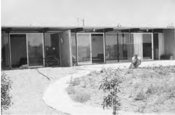
The Bobertz residence in the college area, designed by Craig Ellwood in 1953. Note the floor-to-ceiling glass. The exposed wood beams and columns carry the roof load allowing for open walls of glass. Courtesy of Gerry Bobertz.
