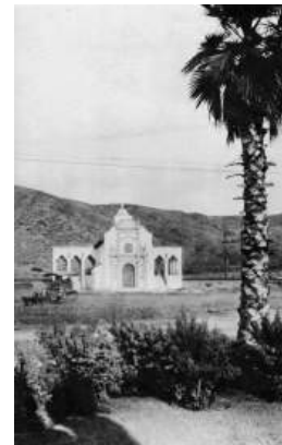
Figure 8 San Carlos Substation, Courtesy of the San Diego Historical Society
