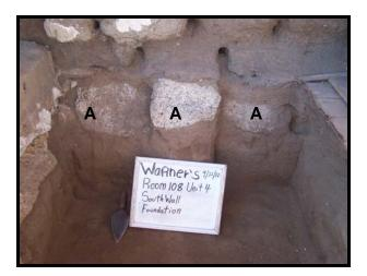
Figure 28: Angular granite fieldstones in the north wall footing of Room 101 (A), as seen in the south wall of Unit 10-4 Room 108. These are typical of the angular granite stone used throughout most of the foundation of the Central Wing.
