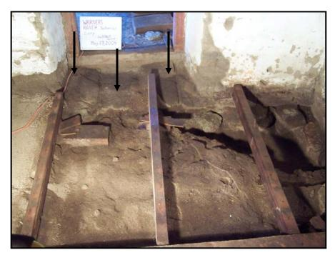
Figure 42: Entry Room (101) Block excavation Sections 2 and 3. The badly worn lower earthen floor and blocks in the door way can clearly be seen.
