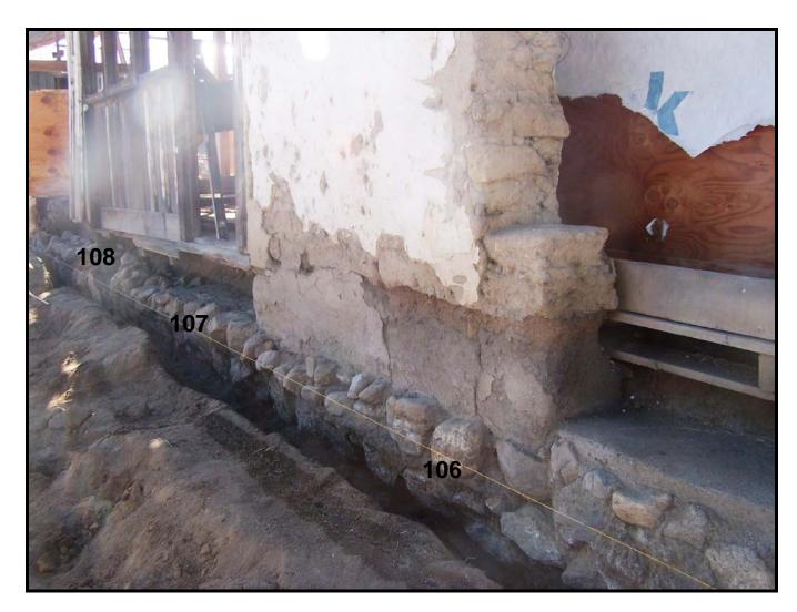
Figure 76: North wall foundation of the North Wing exposed in the restoration construction trench along the northern edges of Rooms 106, 107 and 108. The segment at lower right was capped with concrete during stabilization activities in 2004.
