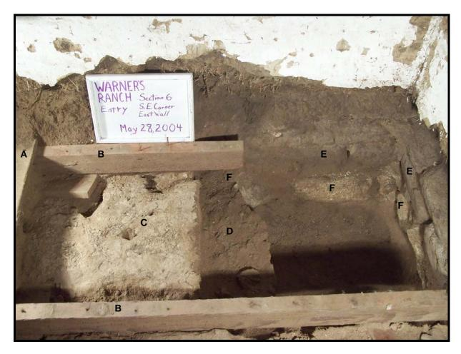
Figure 38: Entry Room (101) block excavation Section 6 following excavation of the northeast corner, looking east. A portion of the far sleeper has been cut off to allow excavation access. Note (A) the present wooden floor board, (B) sleepers, (C) upper earthen floor, (D) lower earthen floor, (E) adobe blocks at the base of the wall, and (F) a single course of field stones underlying the wall.
