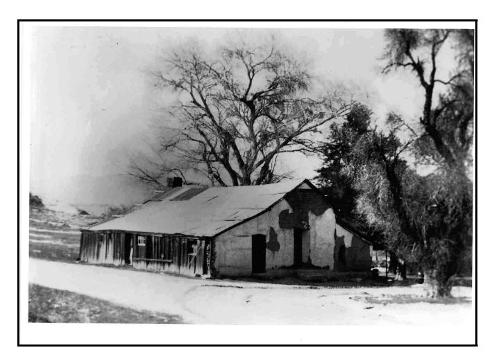
Figure 14: Ranch House at Warner's Ranch around 1935. Note the decayed white wash, weathered siding on the south side, and patches on the roof (San Diego History Center).
