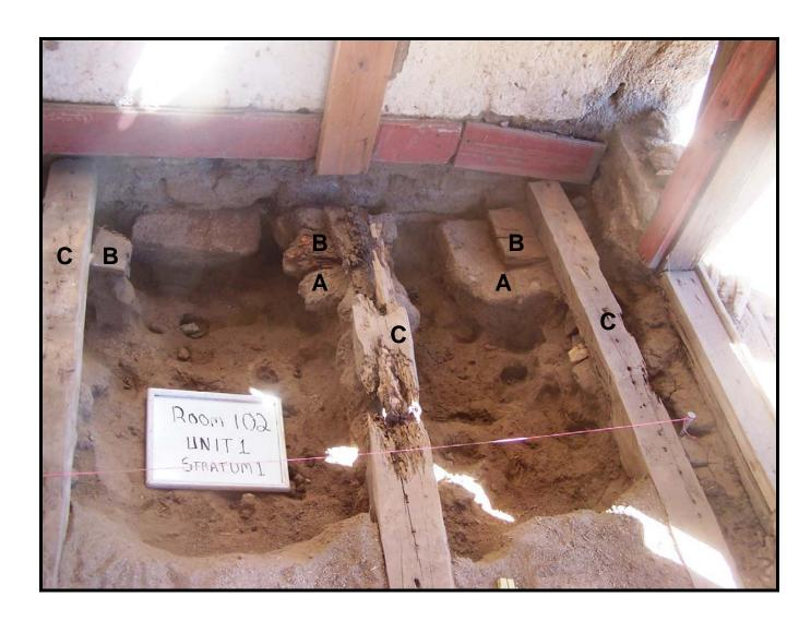
Figure 61: Unit 10-1 excavated to 12 inches below surface. Note the large number of rodent burrows and the adobe blocks (A) supporting wooden boards (B), set under the floor sleepers (C).
