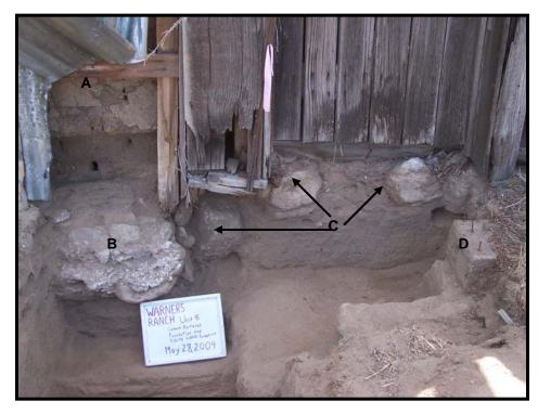
Figure 98: Unit 04-8, showing the adobe blocks of the west wall of the Central Wing (A), lime mortared cobble facing on the foundation of the Central Wing (B), and the remains of the cobble foundation for the original adobe wall on the west side of the South Wing (C), and wood support for the late 19<sup>th</sup> century addition (D).
