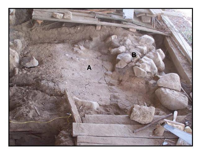
Figure 88: An area of the original porch cleared of debris. Note the hard packed earthen surface that appears to have been laid as a mud slurry (A) and the shallow cobble footing along the north edge (B).
