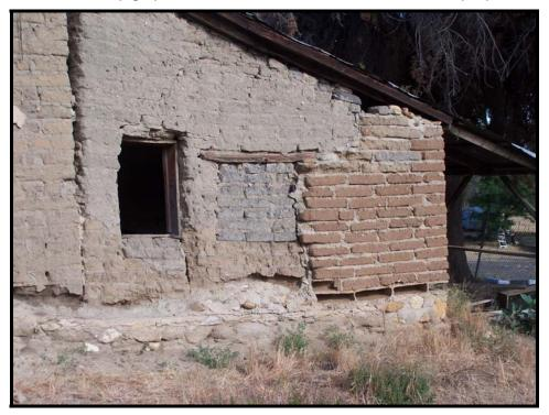
Figure 27: Multiple phases of construction can be seen in the east wall of the North Wing.
