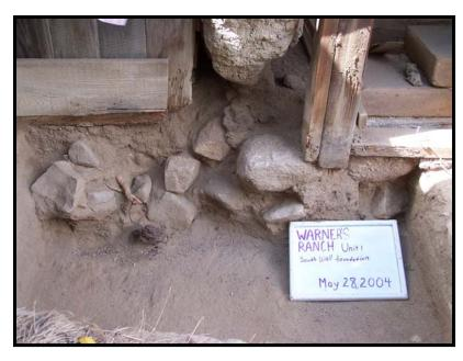
Figure 54: Cobble foundation in Unit 04-1. The west half (left) is badly disturbed while the eastern portion remains intact.
