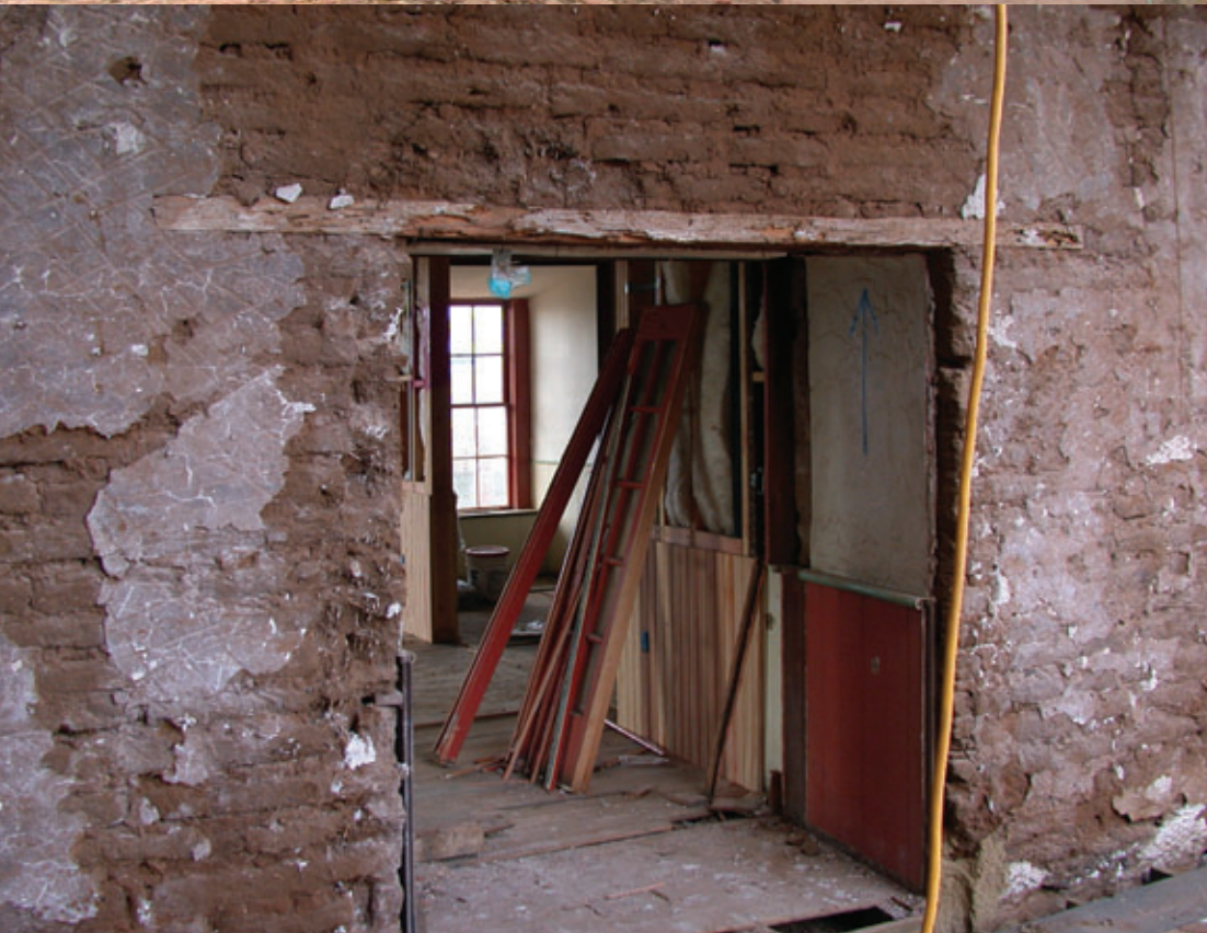
Top The courtyard side during restoration shows the original Bandini adobe walls and the second floor with its original 1869 siding. Bottom The doublewide doorway from Bandini period with original lintel, looking into the dining room with Seeley period wainscot visible. Photos by Bruce Coons
