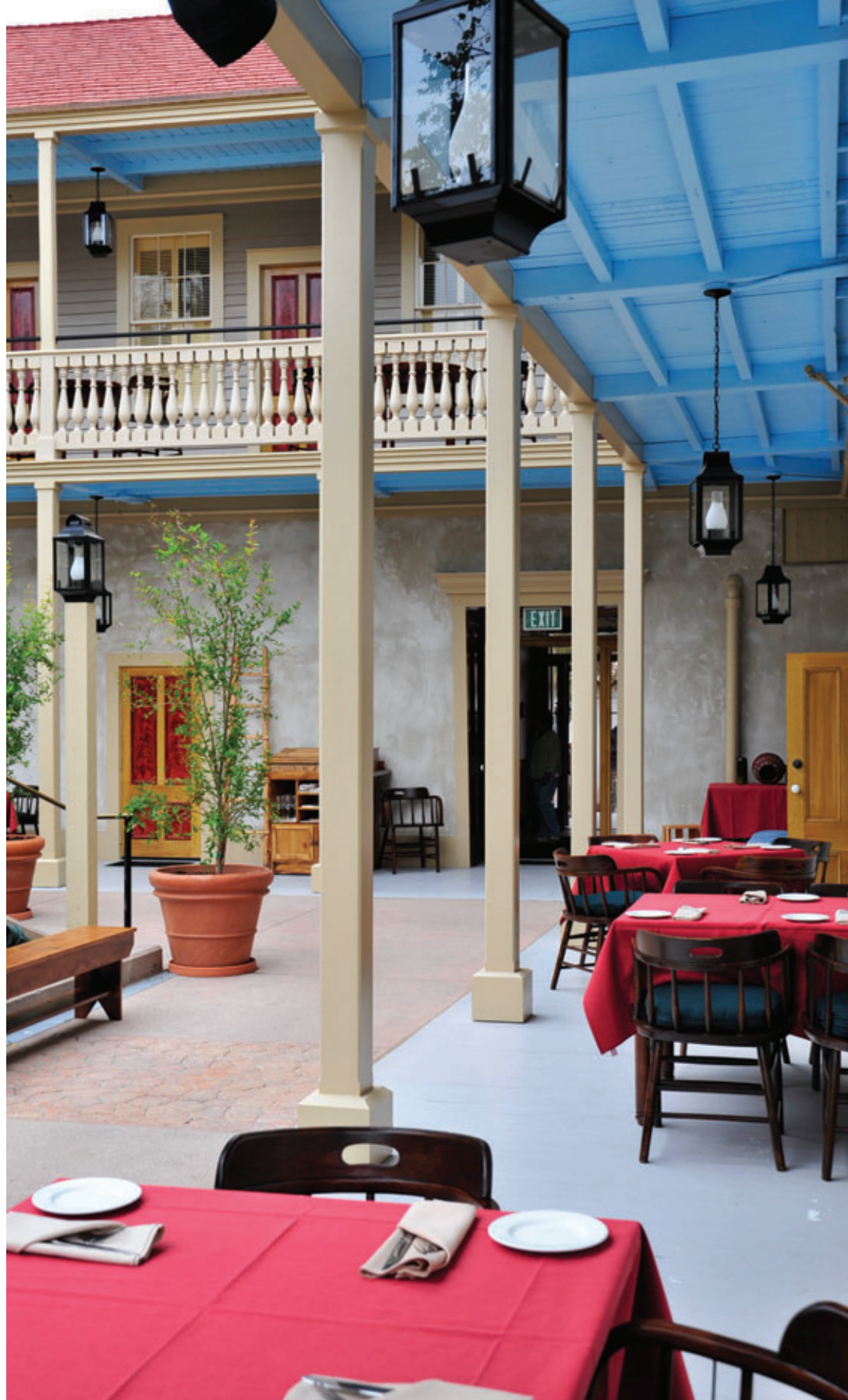
Above The courtyard after restoration, still lacking the final rose beige coat of scored plaster on the first level. The original 1870’s paint colors on all woodwork. Photo by Sandé Lollis
