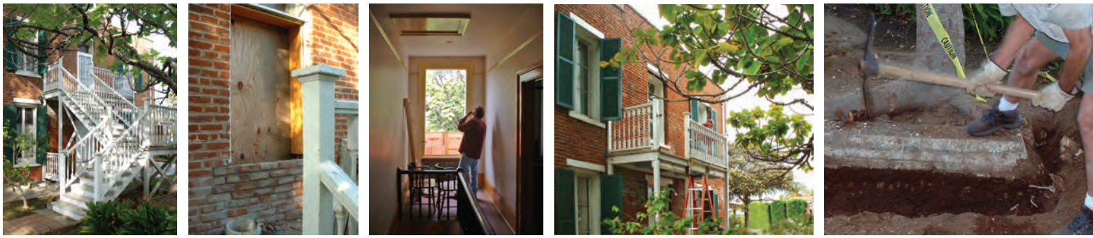
left to right Stairway and door added in the 1960s, photo by Sandé Lollis; restoration begins with removal of stairway and replacement of French window and brickwork, photos by Dean Glass
