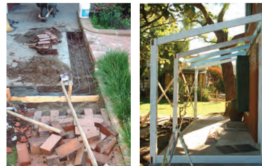
above Thomas Whaley's own drawing for the remodeling of the Whaley house, the kitchen is shown by the 12' x 8' space on the back porch. Dated 1868; bottom left to right Porch reconstruction underway, photos by Dean Glass; final photo Nearing completion of the back porch and kitchen, photo by Sandé Lollis
