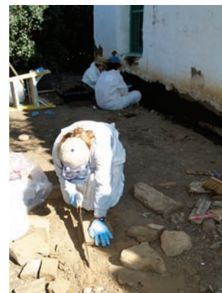
Teri Delcamp uses a hand saw to cut an adobe brick to size
