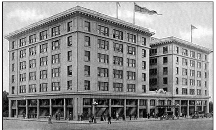
Built in 1914, historic Hotel San Diego is slated for demolition to make way for the Federal Courthouse project.
